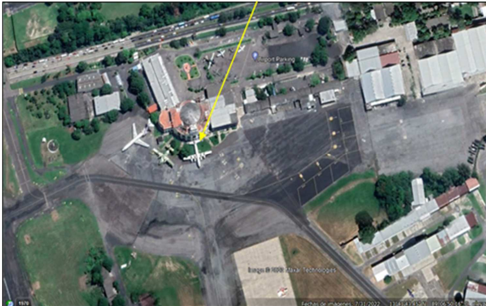
New passenger service area
